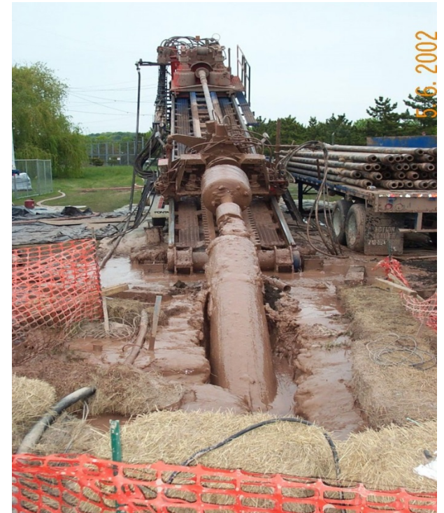
HDPE Casing Pull-Back
